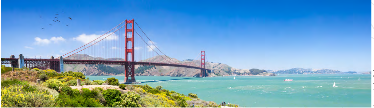
Golden Gate Bridge in San Francisco
